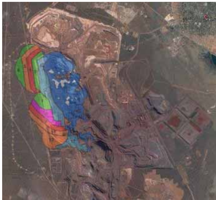
G50 and G80 mining areas in the north pit of Sishen mine
